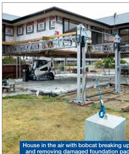
House in the air with bobcat breaking up and removing damaged foundation pad
